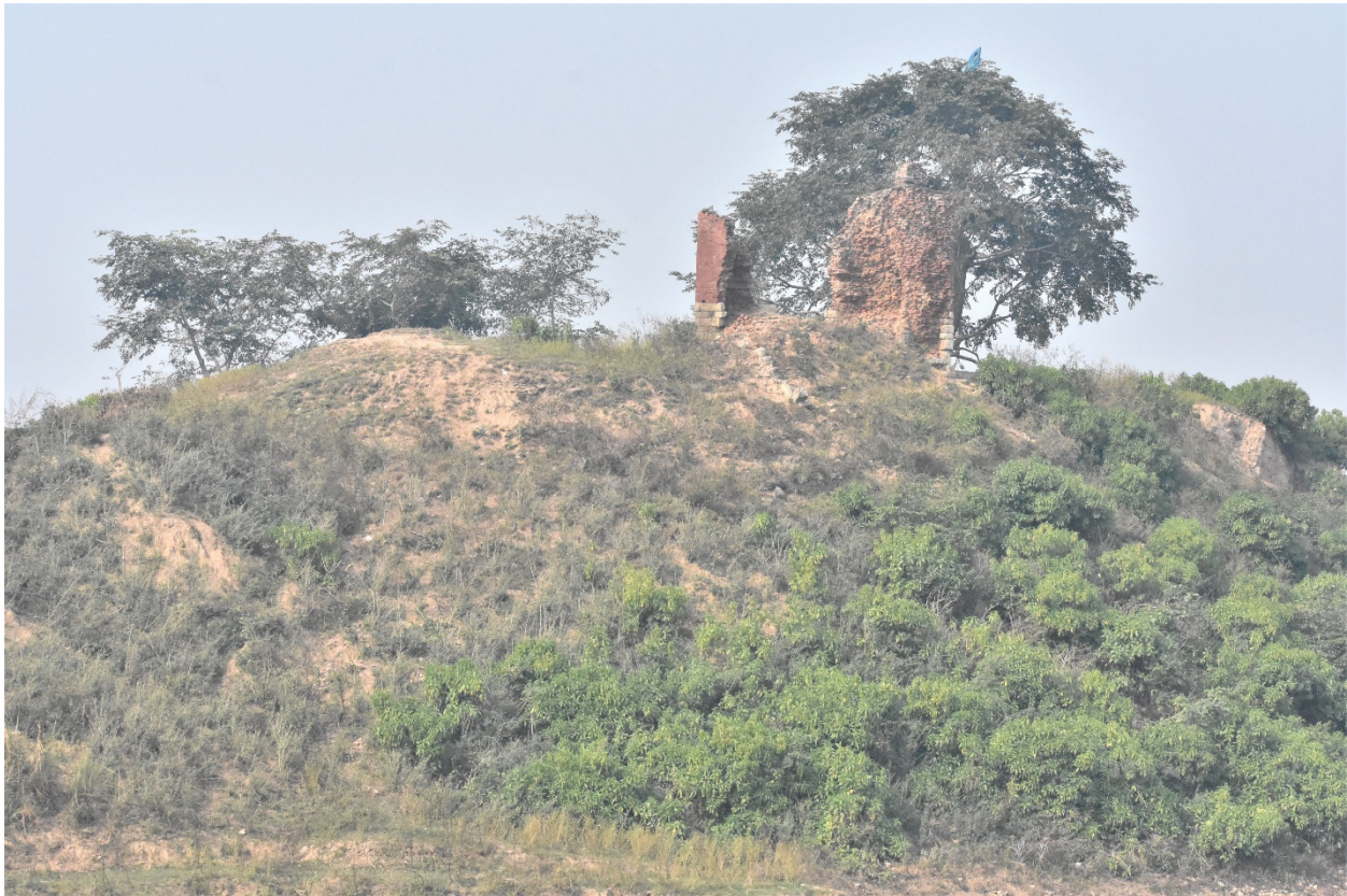
Image 44 : Lateral Bank Erosion Affecting A Heritage Site In Bhojpur Area Of Farrukhabad Distt.
