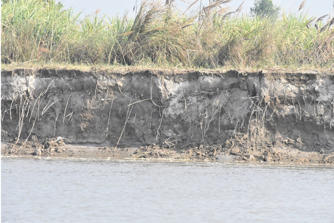
Image 45 : Ganga River Bank Erosion As Observed Near Sukhania In Shahjahanpur Distt.
