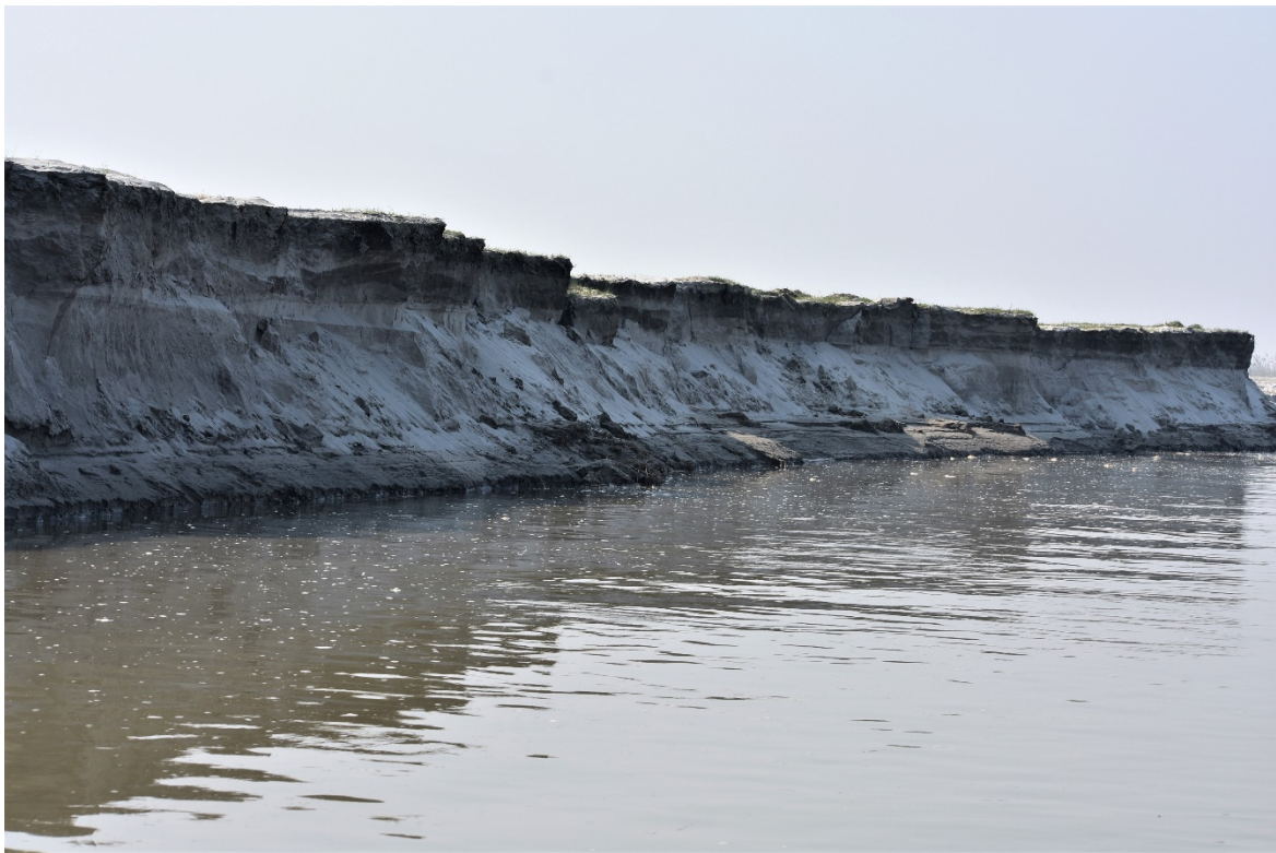
Image 46 : Ganga River Bank Erosion As Observed Near Katridharampur In Farrukhabad Distt.
